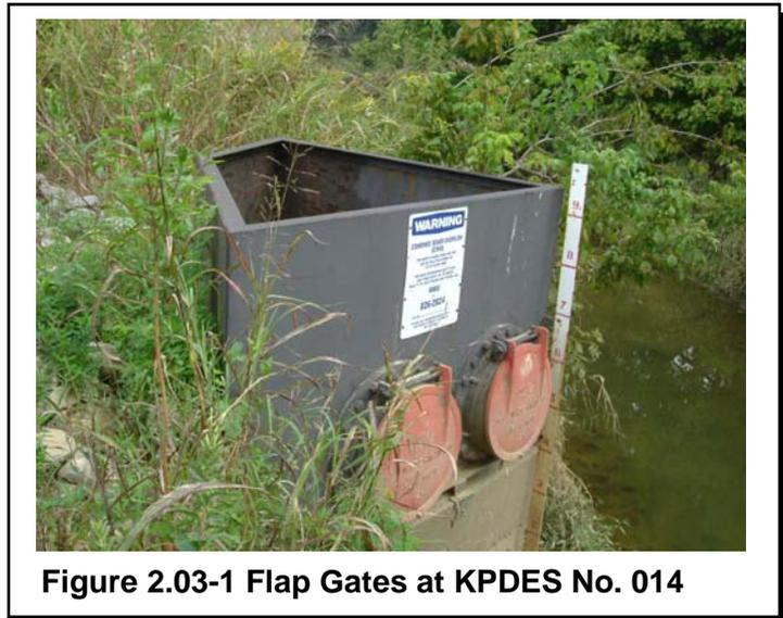
**Figure 2.03-1 Flap Gates at KPDES No. 014**
